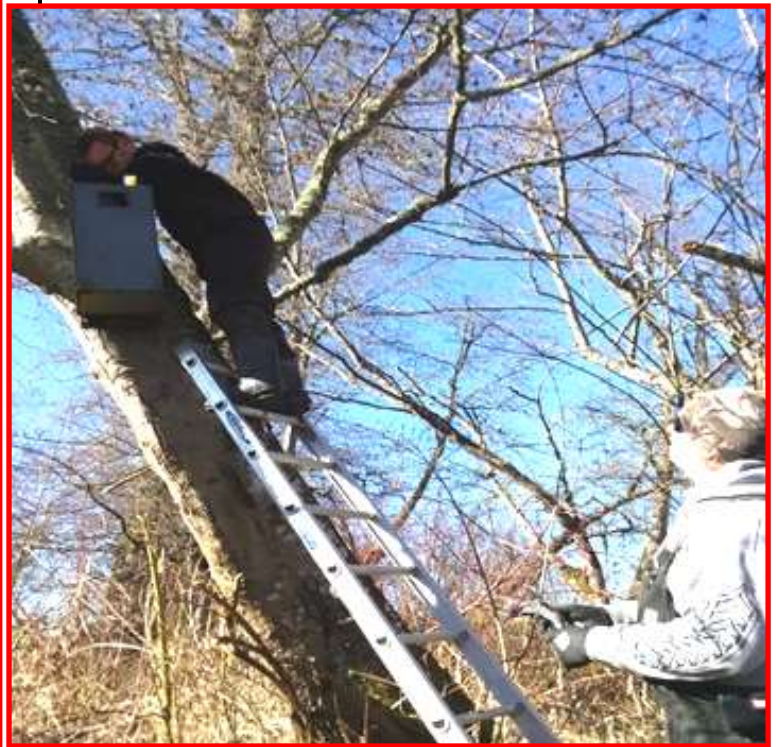
NW Chapter Members, Avery Miller and Mike Rathvon at Milltown Island repairing and installing wood duck boxes.
